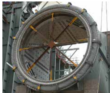
Installation of Combine-X on diffuser.
