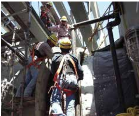
Fabric expansion joint installed over the manifold.
