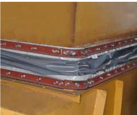
KE-Flex installed in an air duct.
