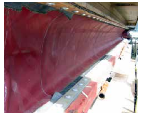
Fluachem Fluoropolymer installed in a vertical duct.
