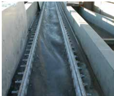
Fluachem Elastomer installed in a horizontal duct.
