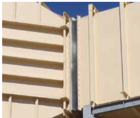
Acouseal installed in gas turbine air inlet.
