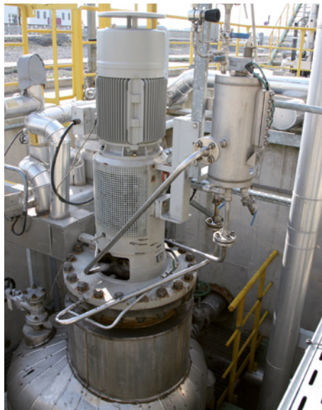
Agitator seal with TS-system
